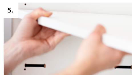
5. Move the shelf down from above until the positioning pins lock into place in the counterpart
