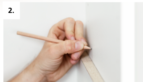
2. Mark the milling axis from the shelf to the desired position on the sides of the cabinet
